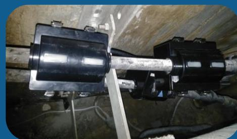
Tolenoid™ C power supplies attached to the cross-bonding ground cables in the underground power vaults, powering the sensors and communications modems
